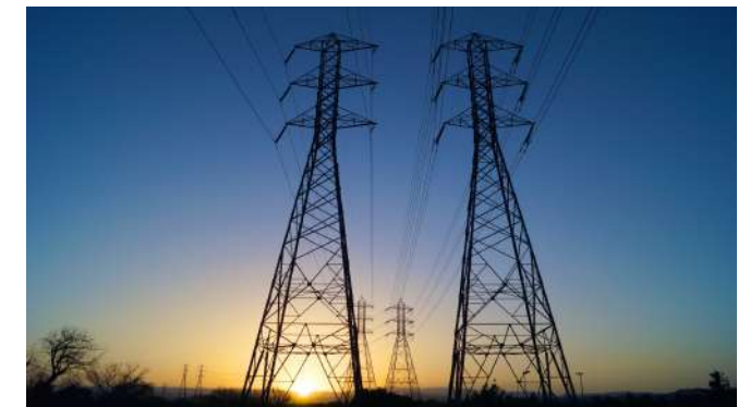
power grid analysis
